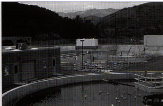
The Ojai Valley Sanitary District 3.0 MGD tertiary treatment facility is located between Ventura and Ojai in the south coast region of California.
